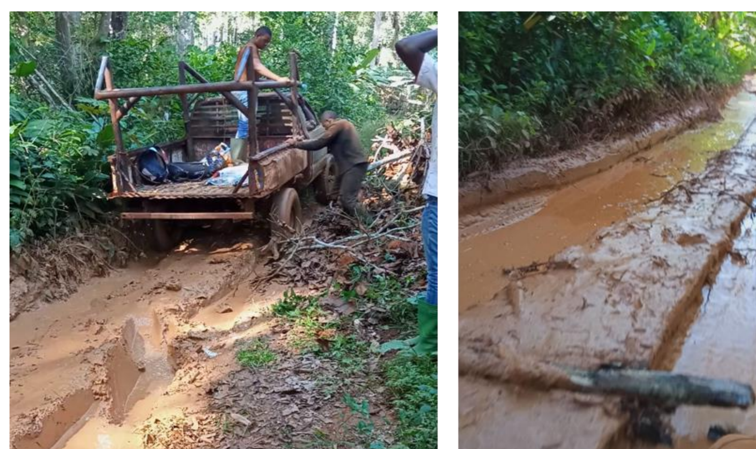
State of practicability of roads serving production basins
